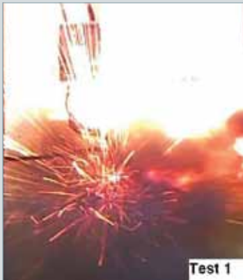
Figure 2. During test. Heater elements were vaporized and contacts solidly welded. Type 1 performance.
