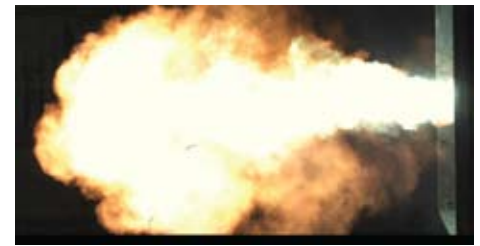
Arc fault delivered to a circuit without fusing.
