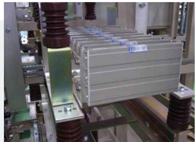
Figure 4: Semiconductor fuses rated at 10kV 1000A with low inductance
